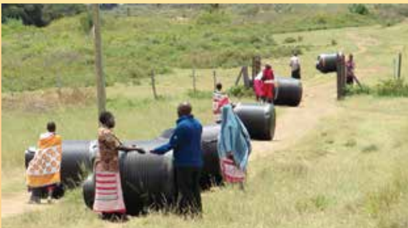
Suswa Water Tank project
